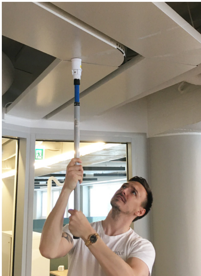
STRATUR'S EXPERTS install beacons at Aktia's new HQ in Helsinki, Finland.
